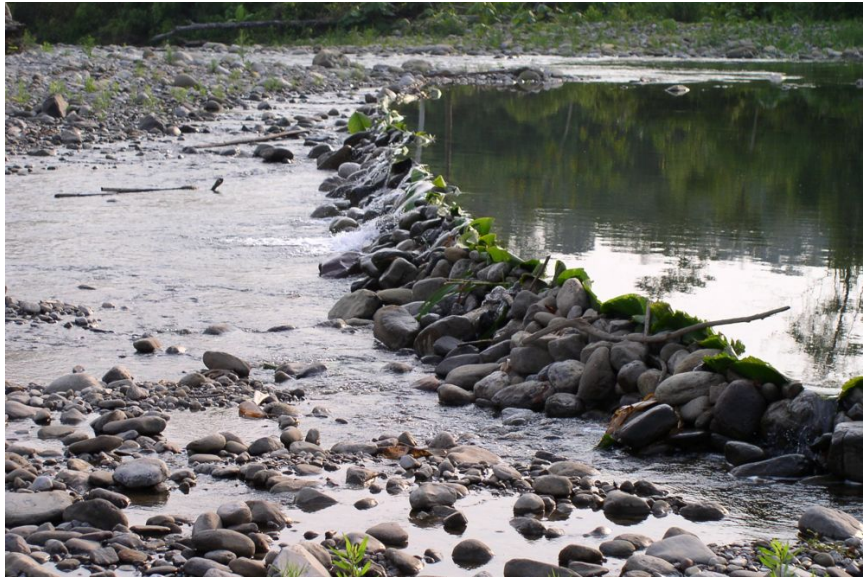
Figure 2.10: In the dry season months when the river level was already low, residents of Montetoni often built fishing dams across a section of the river, as shown here in 2004. Rocks were arranged and then leaves placed along the upriver side to seal the gaps between the rocks. The purpose of the dam was to create shallow areas in which individuals could easily hand-gather or arrow-pierce fish visible in the crystal-clear waters.
